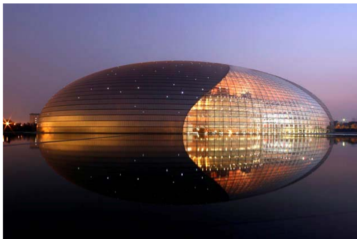
National Grand Theatre Beijing (Architekt Paul Andreu)
